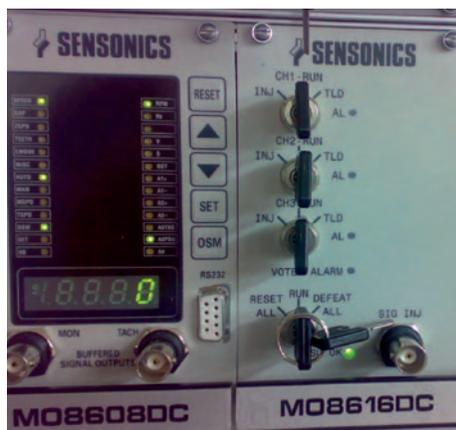
A wide range of Sensonics equipment was selected to provide the essential function of monitoring and protecting the condition of the key operational rotating plant. Original monitoring systems replaced included the turbine supervisory equipment and vibration
