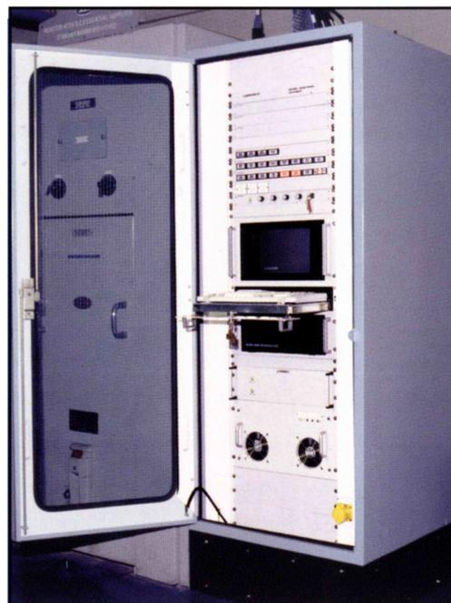
The seismic detectors provide a seismic event alarm at the operating base earthquake (OBE) level that should be set above the anticipated background vibration level. However, to protect against spurious trips, the following precautions are taken.
